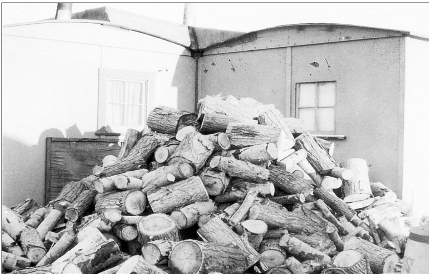
A wood pile sits ready to heat an office in Wheeler, near the Fort Peck Dam construction site. Date unknown.
